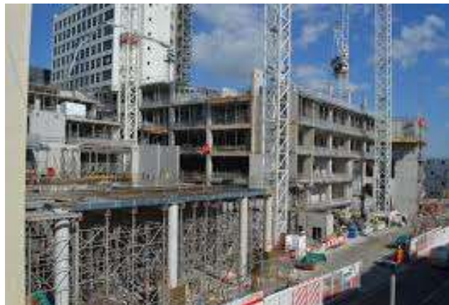
Fig. 1. The hospital construction site (Source: Google Images, 2018)
